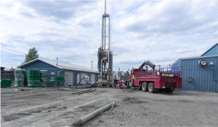
Vertical boreholes of the GeoExchange field go down to depths of 500 ft (~150 m).
